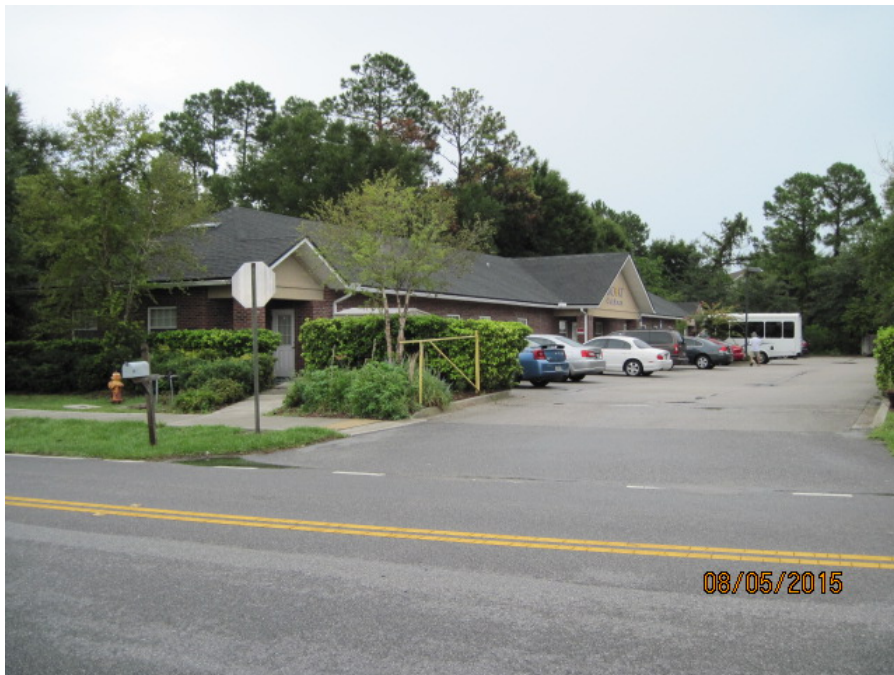
Existing commercial office across Cortez Road
